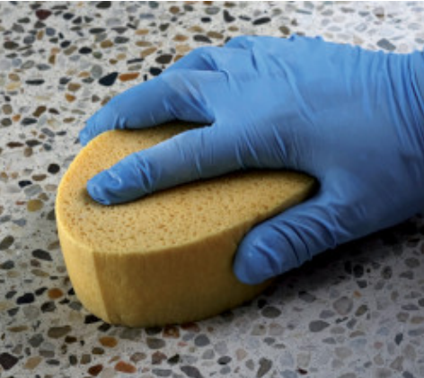
Damping the surface with a sponge
