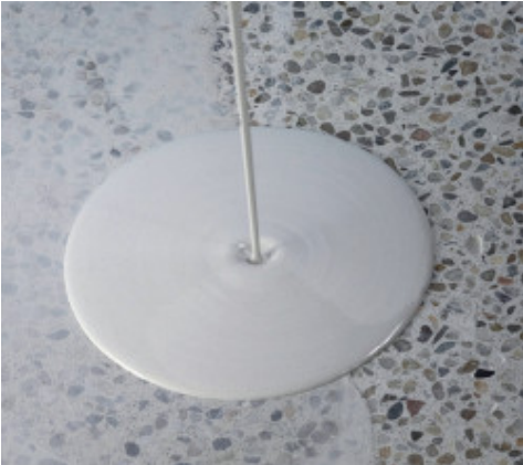
Application of Ultratop Stucco
